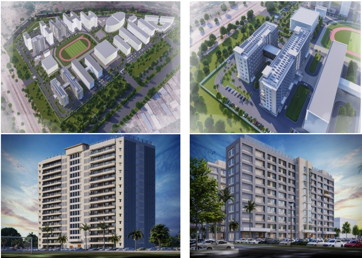
Figure 1: View of the under Development NIT Delhi Campus
